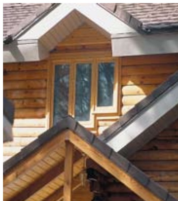
Enclose eaves and soffits.
